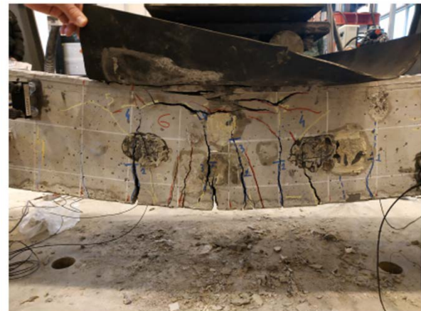
Figure 5. Crack pattern at failure of beam T3a.
