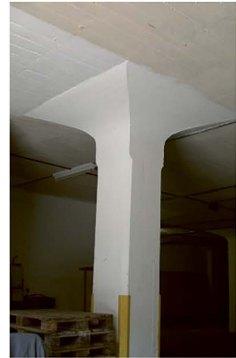
Figure 12. (a) normalized punching shear resistance as a function of the effective depth according to the Swiss codes since 1956 ( f_{ck} = 30 MPa, c/d = 1.25 , \rho = 0.75\% ); (b) mushrooms slabs with capitals according to Maillart and (c) Magazzini Generali at Chiasso Switzerland, 1924-25.
