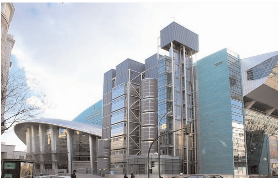
Fig. 18. Torres de Servicios. Figure 18. Service tower.
