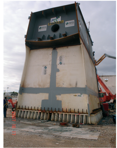
Figura 21. Base. Figure 21. Pier.
